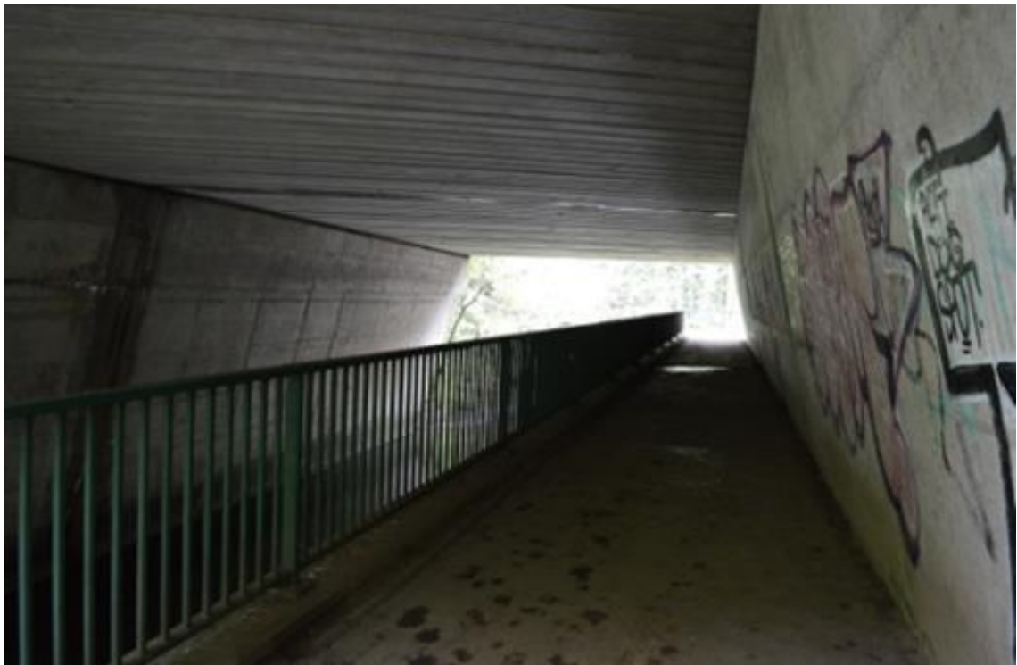
Figure 31. The Bollin underpass beneath the M56 in Ashley; evidence of urban qualities entering in to the river valley, resulting in a forbidding experience for any solo walker (author's photo, 15.10.2015)
