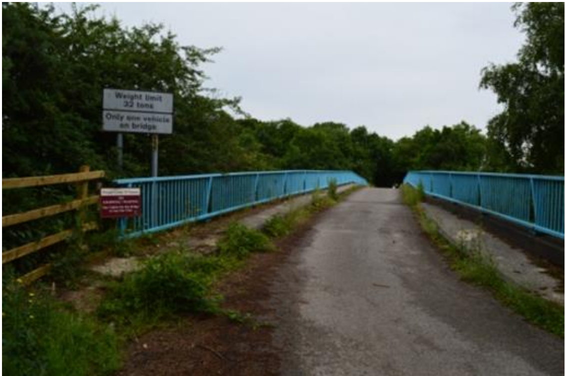
Figure 32. Hall Lane, Ashley, crossing the M56. It is a private road and designated public footpath; cyclists are banned from using it, warned off by signage and asked to dismount by Tatton Estate employees (author's photo, 12.09.2015).
