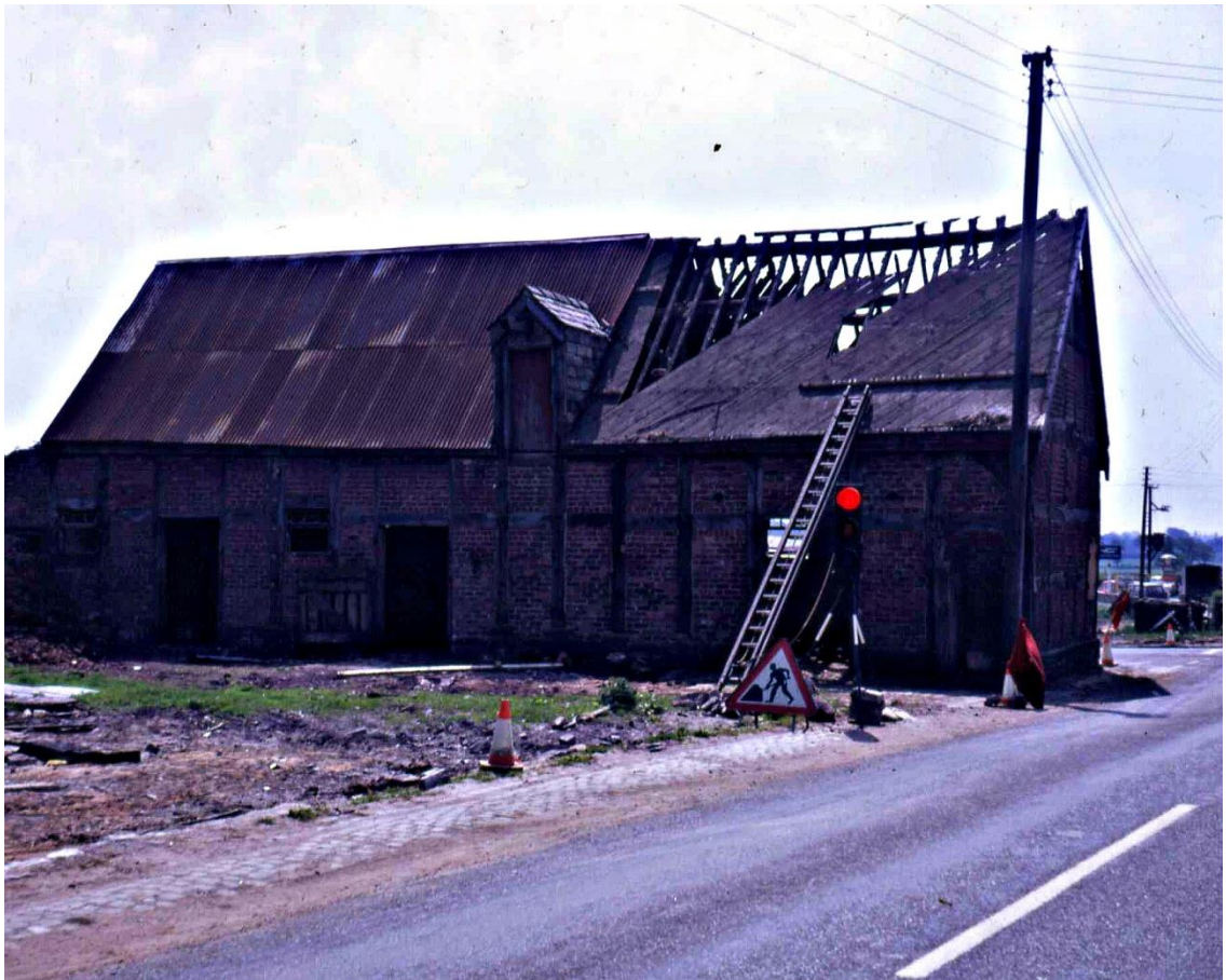
Figure 41. Demolition of end bay of Ashley Barn, 1970, in order for road widening to take place at the centre of the village (photo taken and kindly supplied by Peter Wright).
