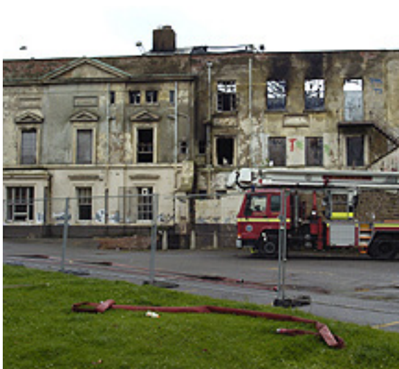
Fig. 99 Central Park fire (2008). Image from https://tinyurl.com/znfsmwd .
