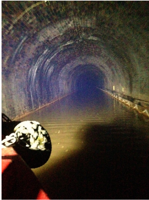
Figure 10. Harecastle tunnel on the Trent and Mersey Canal, Kidsgrove. Photo: Author, 2016.
