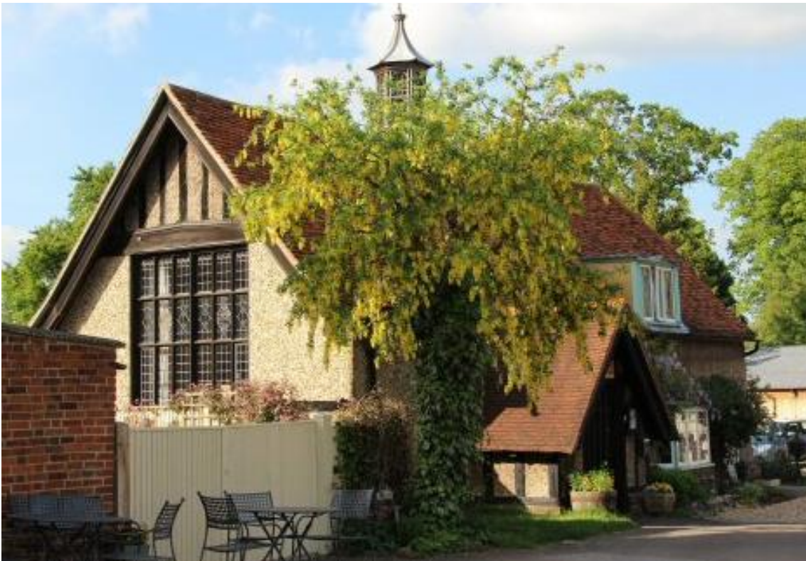
Figure 6.17: Westmill Village Hall, barn conversion by architect Charles Spooner, 1901. Owned by the Guild of St George and administered by the T. and M. Greg Trust.
