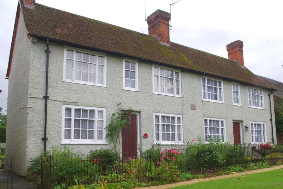
Figure 6.16: Hope Cottages, Westmill, built in 1911. Owned by the Guild of St George and administered by the T. and M. Greg Trust.
