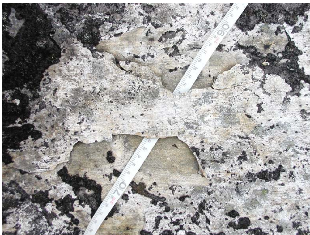
Figure 8. Shallow surface spalling in quartzitic schist.
