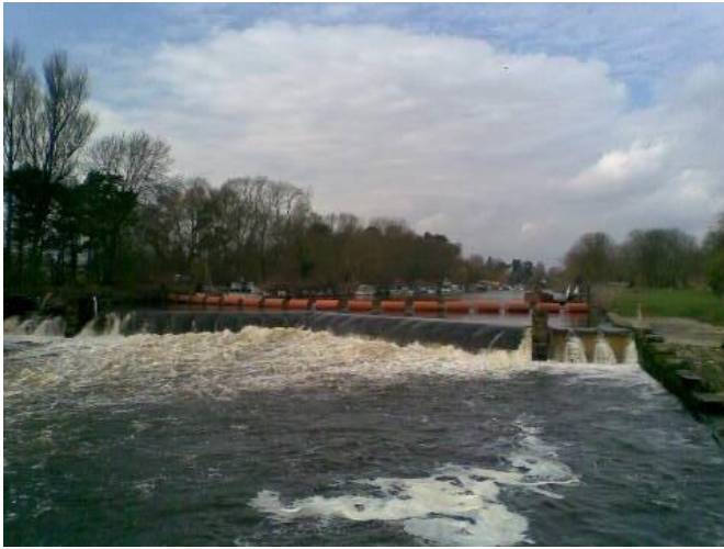
Figure 13: A typical investigation site – weirs on a river in the north-east of England
