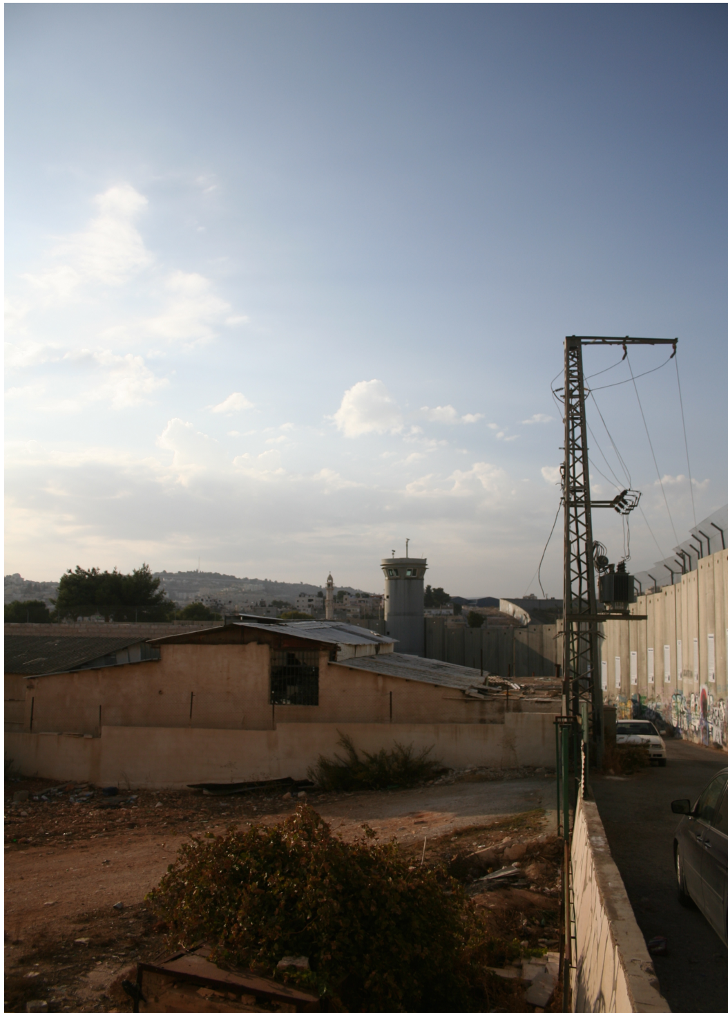
Figure 27: The close proximity of the barrier to Palestinian homes. Figure 28 shows an image of the same portion of the barrier from the other side. The barrier blocks light and space while at the same time, a watchtower overlooks the property too. Photo by Author (2013).
