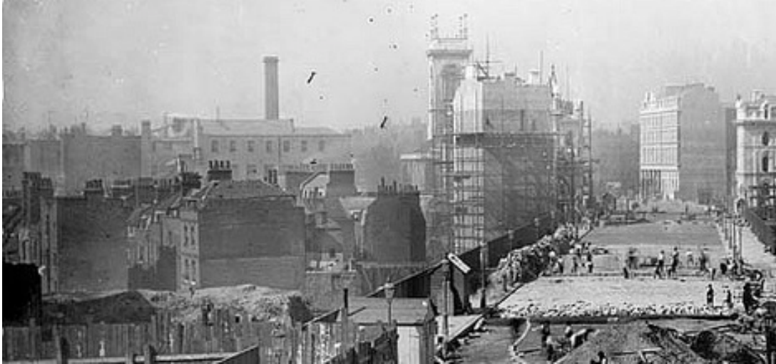
Figure 85: The eastern end of Plumtree Court visible from the nearly-complete Holborn Viaduct, 1869. Illustrated London News .
