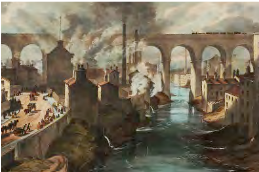
Figure 5.16 'Stockport Viaduct', AF Tait 1848
