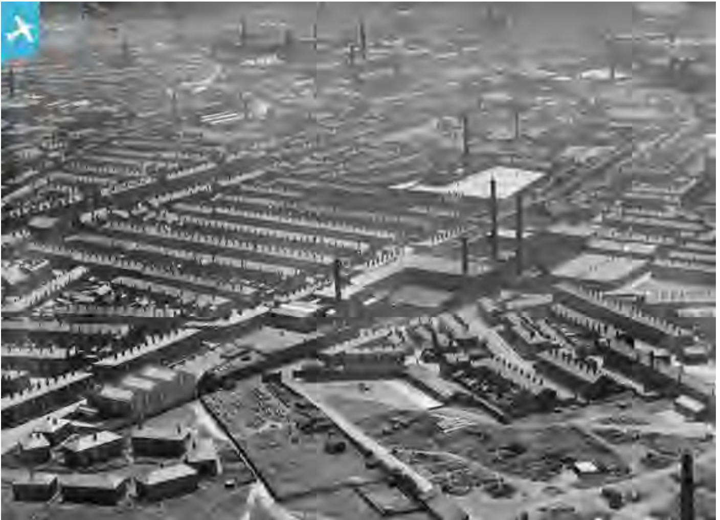
Figure 4.16 Aerial View of Bury, 1933, courtesy of Britain from Above. The image shows Bury, largely unrecognisable in relation to its current layout. The scene is dominated by terraced housing and mill buildings, very little of which still survives.
