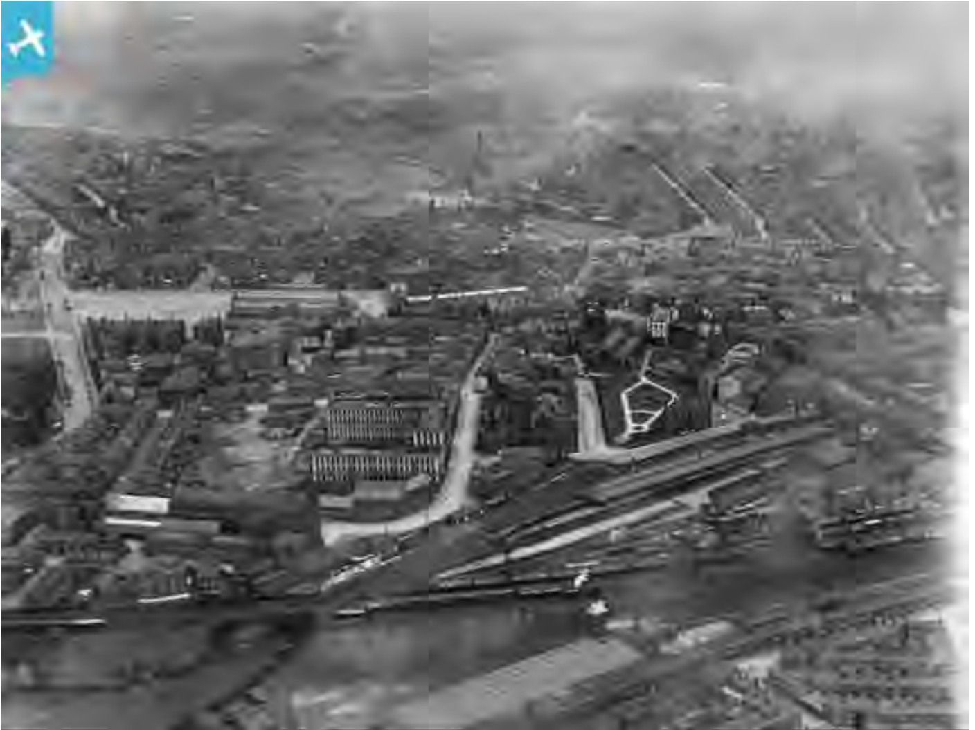
Figure 4.21 Aerial View of Wigan, 1920, courtesy of Britain from Above. The image shows the sprawling character of Wigan with vast rows of terraced housing but also the presence of vast coal pits and wastelands. Transport infrastructures dominate the town.
