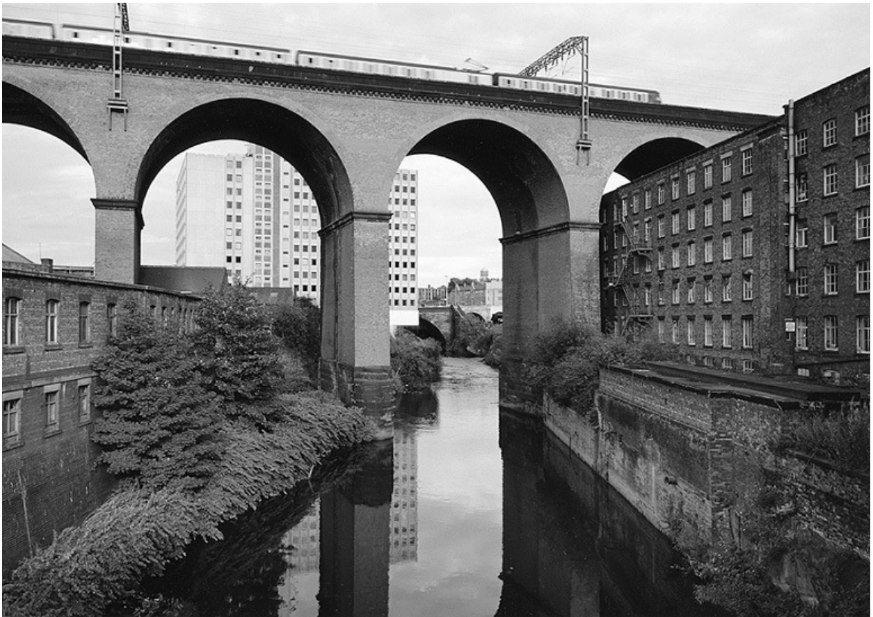
Figure 5.39 Stockport Viaduct, Davies, c.1986, showing the complex built layering of Stockport and elements of deterioration documenting the 'traces' of the town's history.
