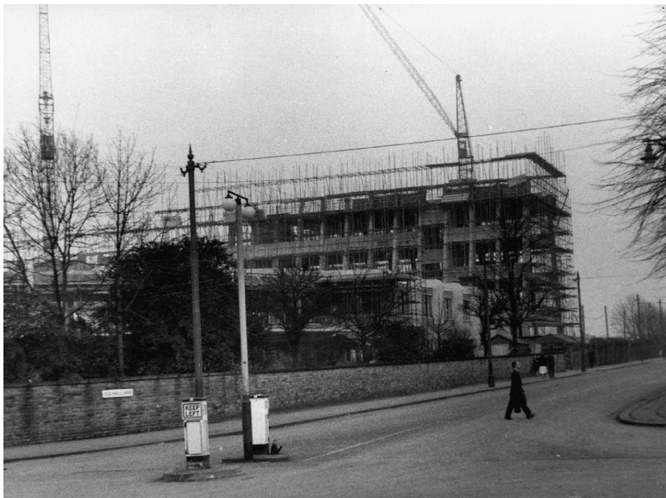
Fig.4.13. Domestic and Trades College under construction 2: post and beam construction evident
