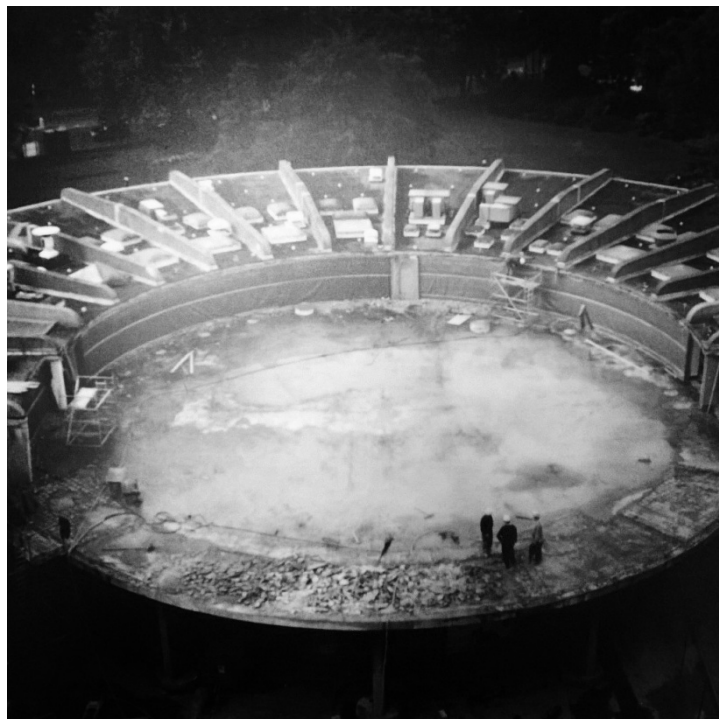
Fig.4.18. Hollings Faculty: assembly hall removed (first floor slab revealed)
