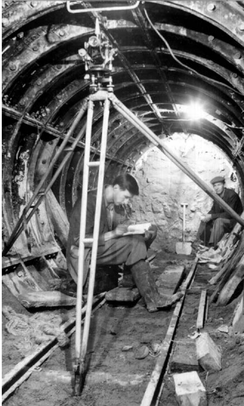
Figure 7. Original photography documenting the construction of the GUTE , dated June 1955. Survey work in progress on one of the smaller cable tunnels. (Source: Photograph by tunnel engineer Patrick Gough. Courtesy of George Coney.)
