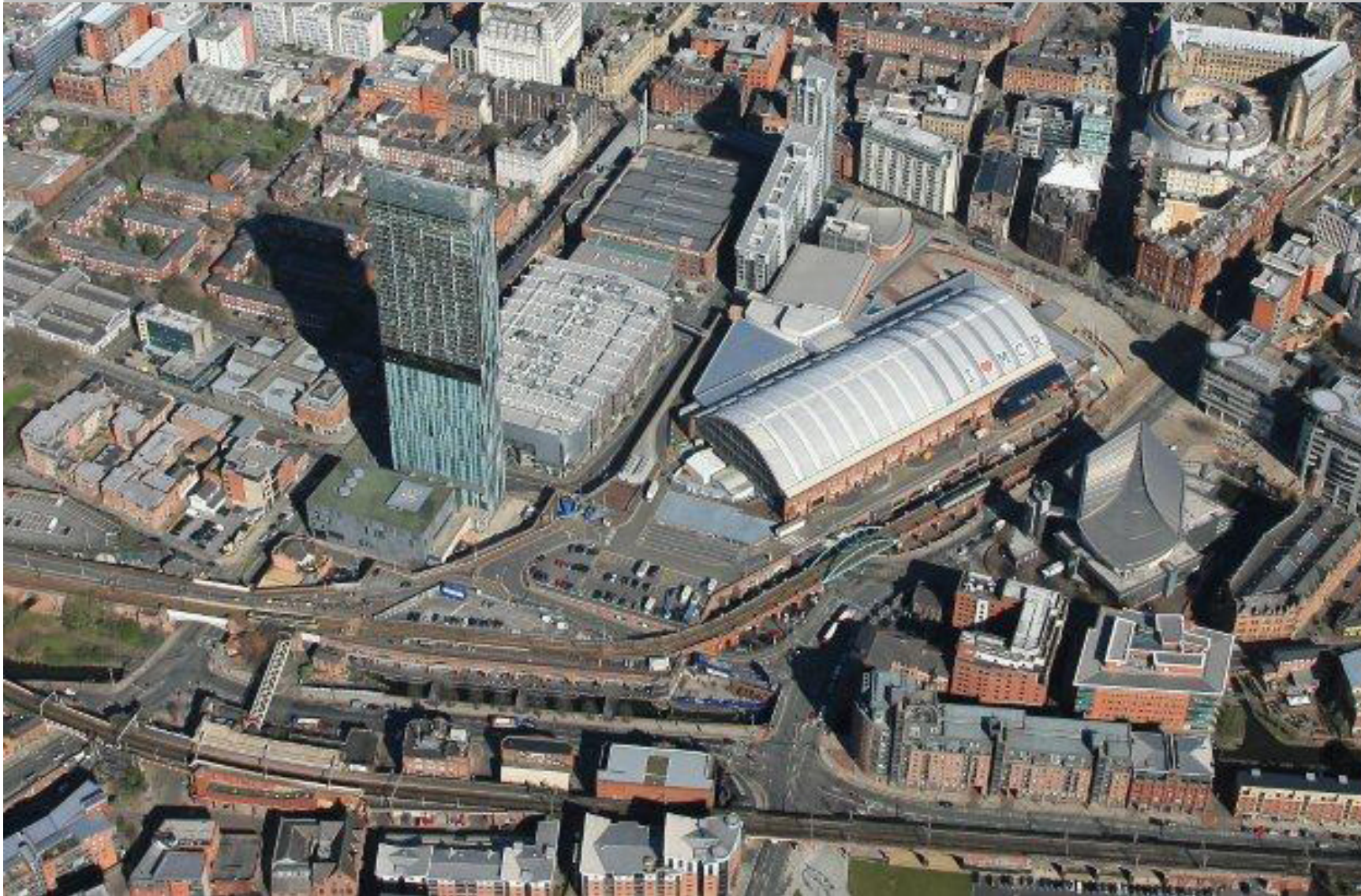
Contemporary aerial view of Central Station site (Source: < http://www.jeffersonairphotography.co.uk/2010/12/aerial-photography-of-manchester.html >)
