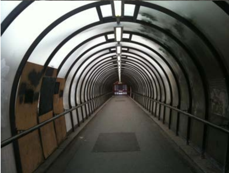
Exhibition footbridge, 1985, Essex Goodman Suggitt for GMC (Source: Author's photographs)
