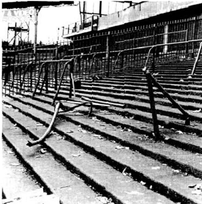
Figure 2.5: Barrier 124A at the Leppings Lane terrace of Hillsborough stadium after the crowd crush. Figures estimate the force required to cause this crush barrier to collapse was in excess of  $8kNm^{-1}$ , or  $8000Nm^{-1}$  [99].
