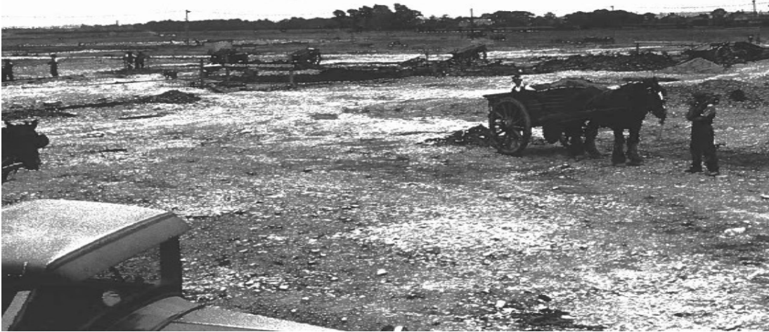
Figure 5.1: Airbus Broughton Foundations Circa 1930's (Source: "Seventy Years of our Broughton"; 2009)
